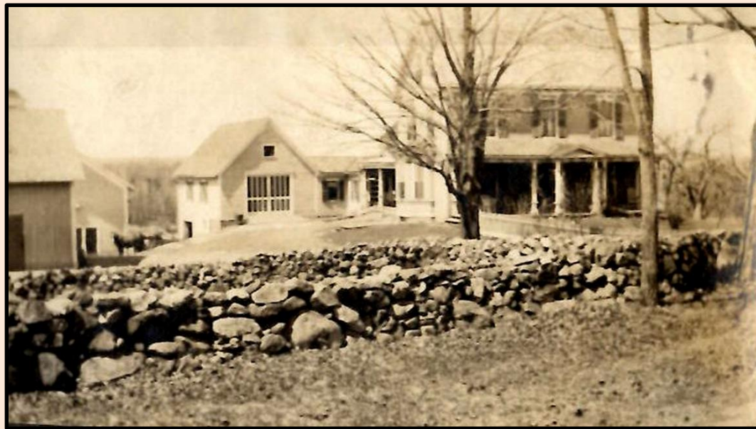
FLAGG FARMHOUSE ORIGINAL LOCATION OF THE KEYES TAVERN WHICH WAS DESTROYED BY FIRE IN 1777 BHSM PHOTOGRAPH COLLECTION
